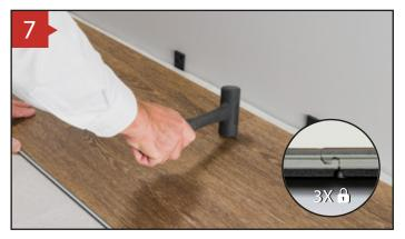
**ENGAGE 3<sup>RD</sup> PLANK ON SHORT SIDE (Part II)** Using a soft rubber mallet slightly tap the joints on the short side to secure. This ensures 3x locking.
