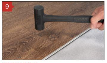
**SECURING PLANKS** As you go, don't forget to use a soft rubber mallet on the short sides to secure the locking.
