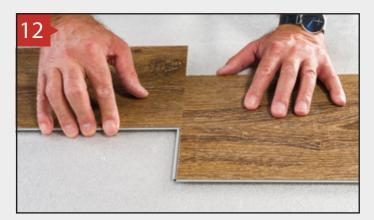
**DISASSEMBLING THE SHORT SIDE** Disassemble the row by sliding apart the planks on the short side.
